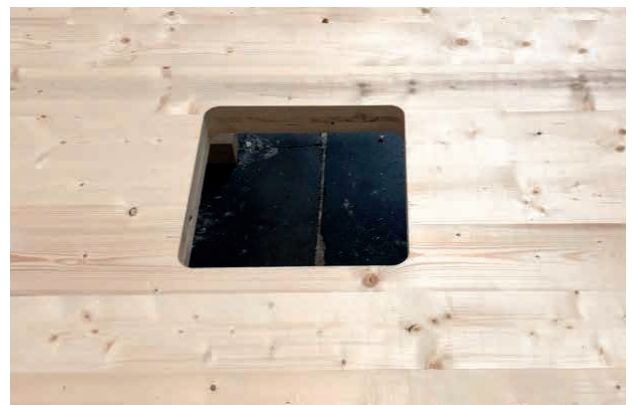
Cut-out, residual radii not removed
