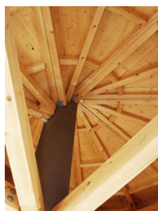
Figure 2.100 – 2.105 The building was completely put together from only eight prefabricated tower segments.
