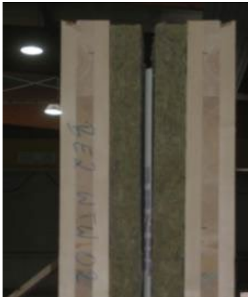
Figure 34: Space of the partition wall filled up with mineral wool (gypsum plasterboard for sound protection reasons)
