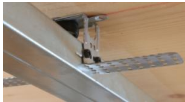
Figure 39: Mounting with decoupled suspension of whip arm, source: Knauf company
