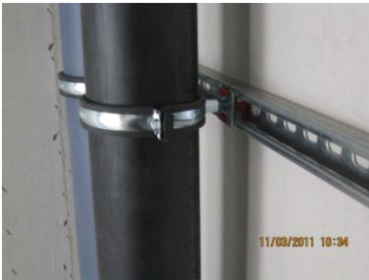
Figure 81: Sound protection decoupling of pipes
