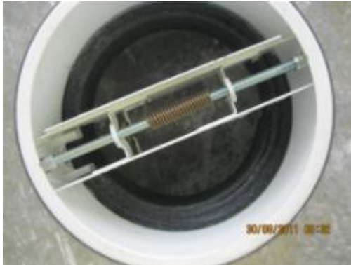
Figure 89: View of a fire protection closure based on intumescent materials with closing element (FLI-VE)
