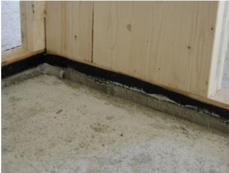
Figure 50: Support detail of an internal wall
