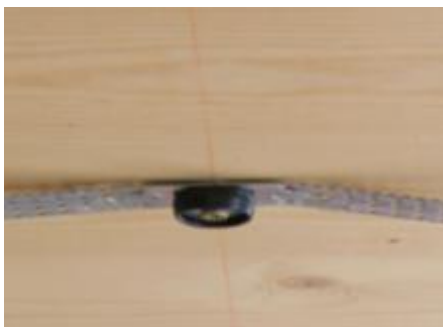
Figure 39: Mounting with decoupled suspension of whip arm, source: Knauf company
