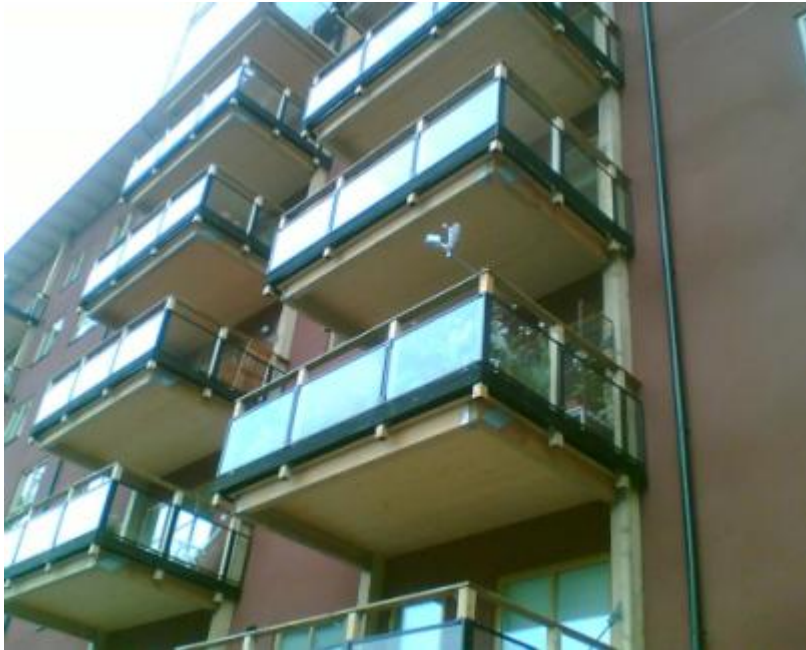
Figure 107: Prefixed balcony construction, source: Stora Enso company
