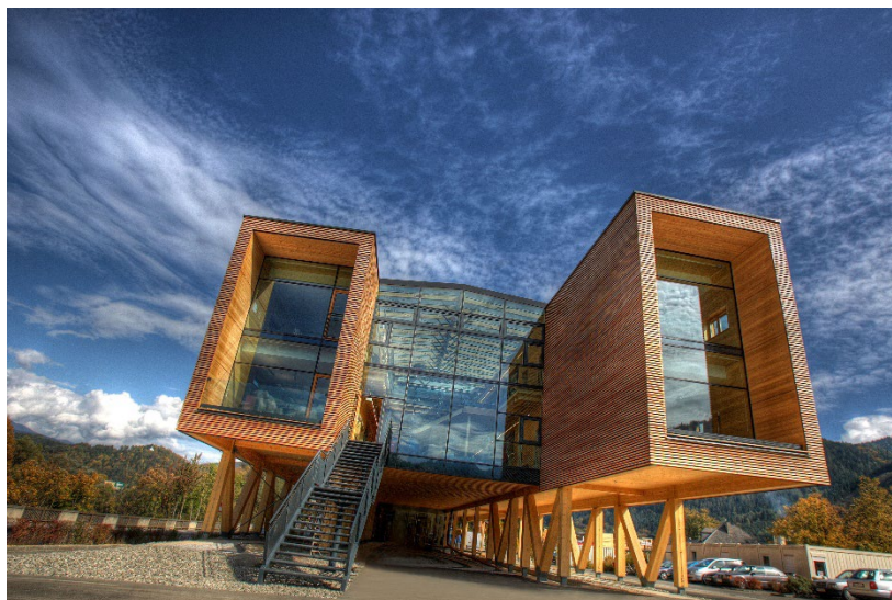
Corporate headquarters Mayr-Melnhof Holz Holding AG, Leoben, Austria (Photocredit: Morgenstern)
